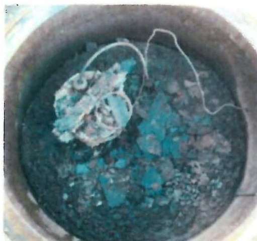
ATG Probe (dyed diesel) – wires are intact
