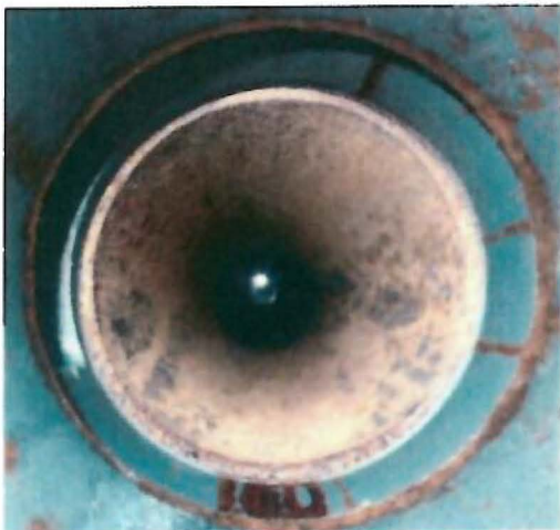
Fill port (plus) – records indicate ball floats for overfill protection
