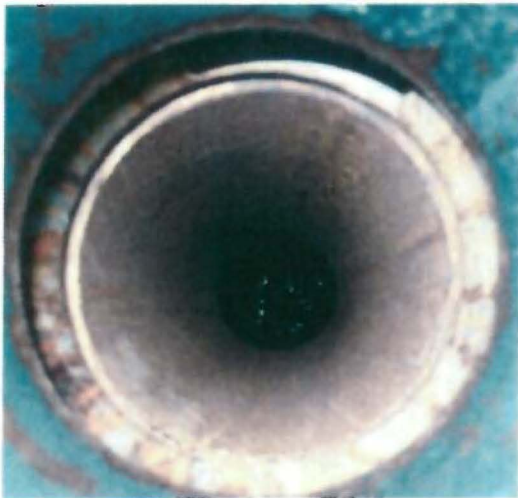
Fill port (premium) – records indicate ball floats for overfill protection
