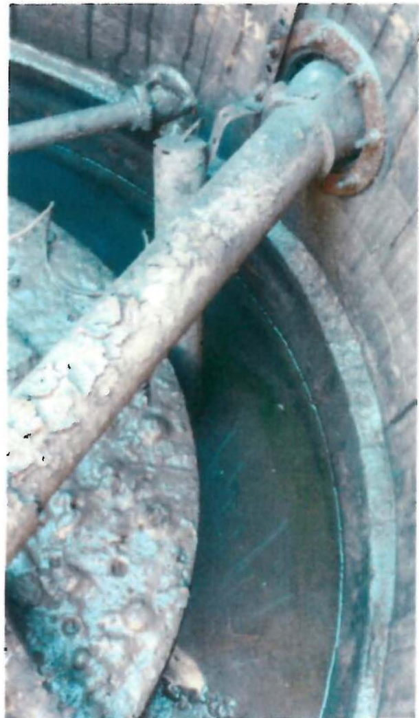
Sump sensor placed higher up in sum, water is visible in sump.
