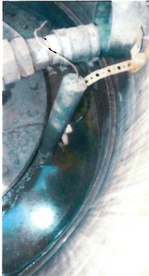
Sump sensor placed higher up in sum, water is visible in sump.
