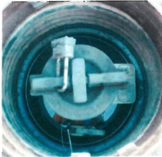
Spill bucket (plus) –generally clean & intact, some water in sump may be result of recent snowmelt
