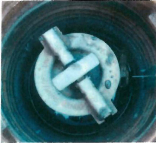
Spill bucket (premium) – clean & intact, some water in sump may be result of recent snowmelt
