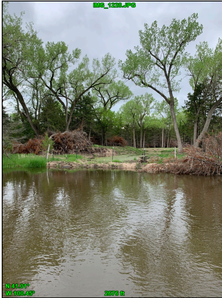
Photo taken from the north side of the channel facing south. The photo shows the area excavated behind the fence line and the berm installed between the channel and the newly excavated channel. There is a plastic culvert (about 24-inch) installed connecting the excavated area to the channel.
