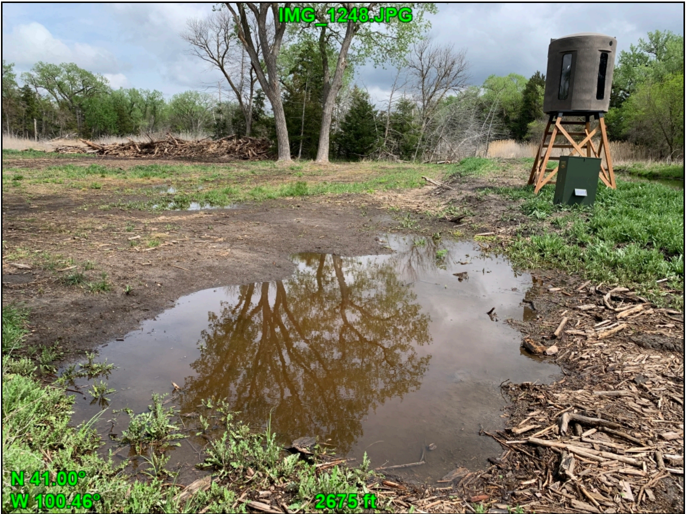
Photo of the berm along excavated channel.
