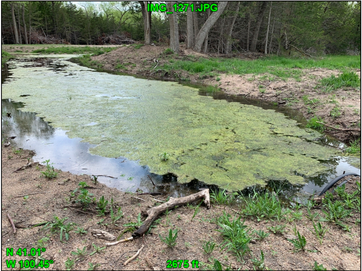
From the berm facing west showing area of excavation.
