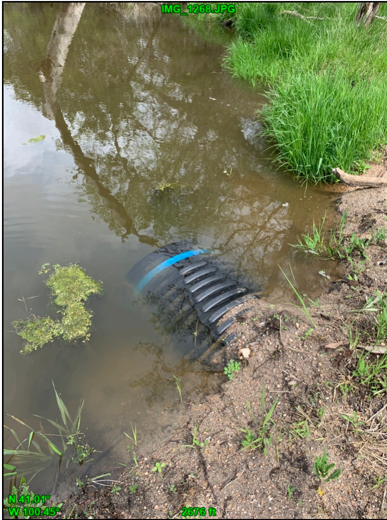
Culvert outlet at Platte River
