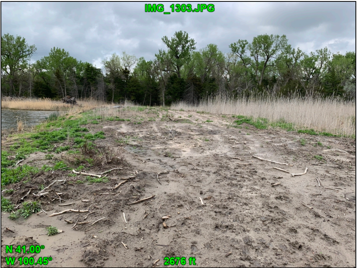
Roadway constructed and crossings installed.
