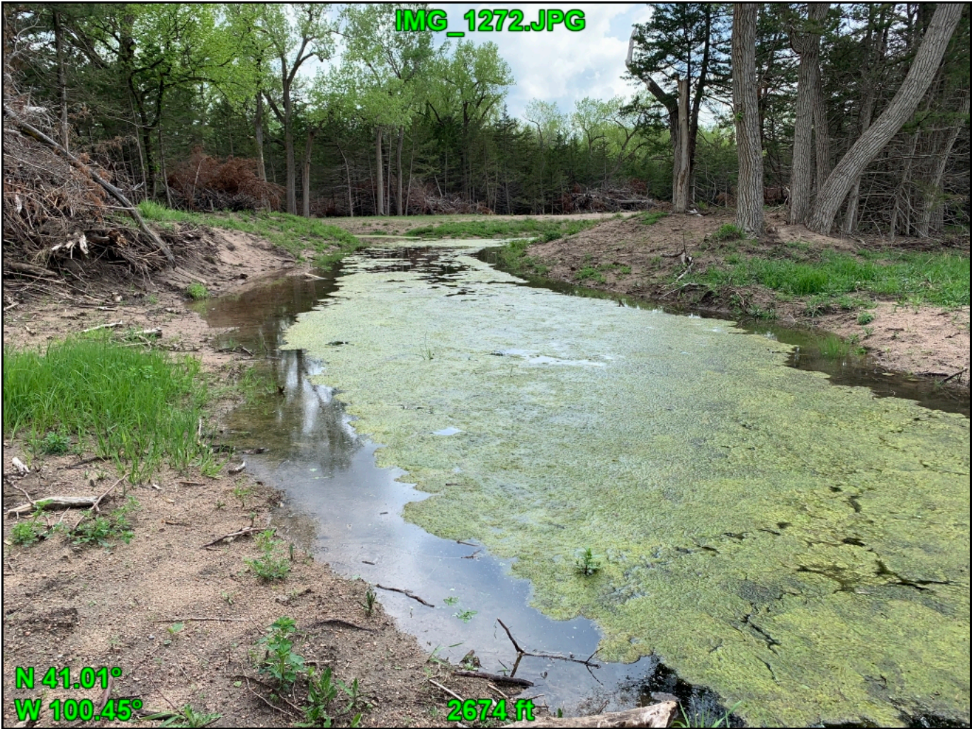
From berm facing south showing area of excavation.
