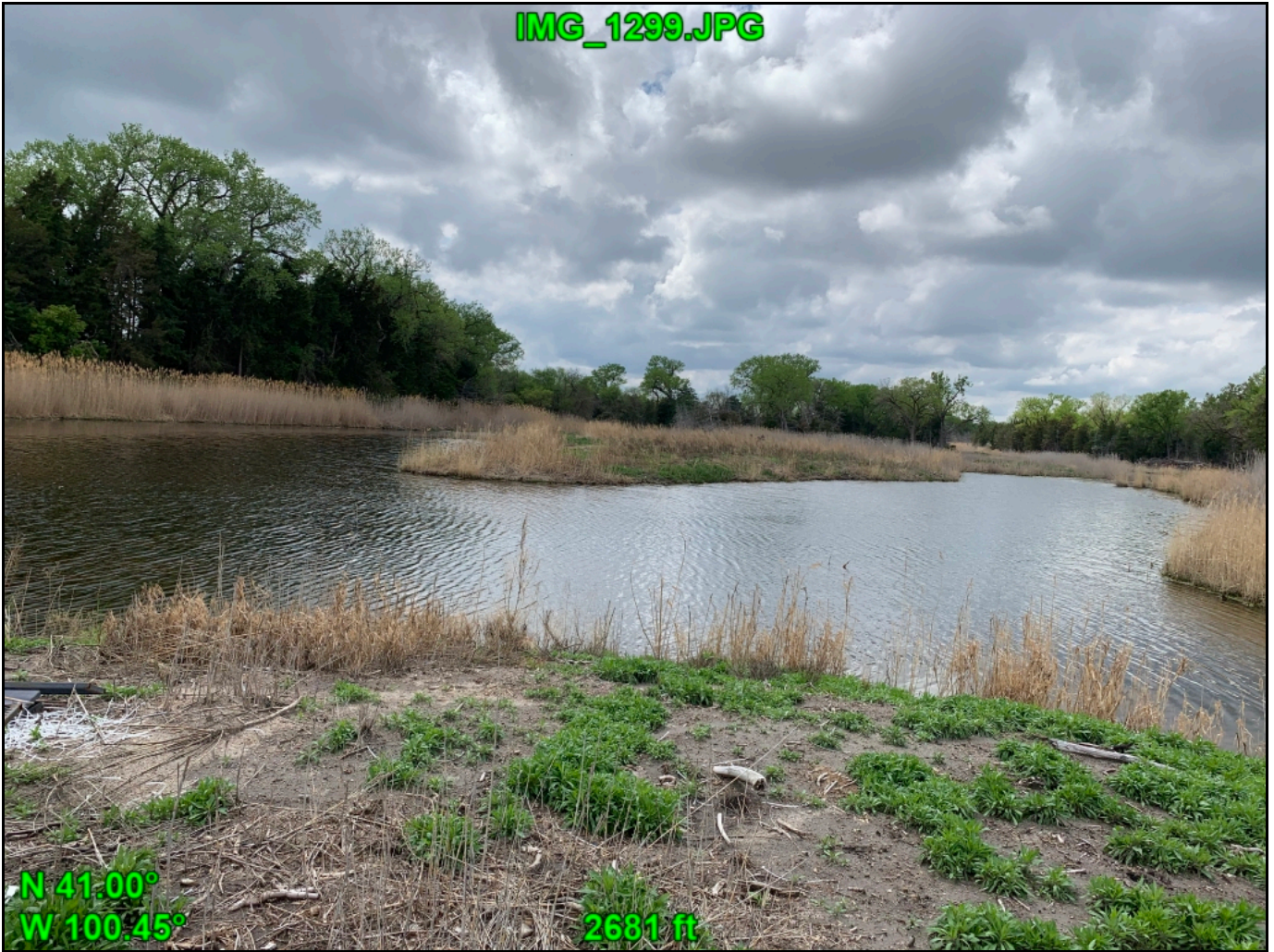
Shows excavated channels west from crossing 3.
