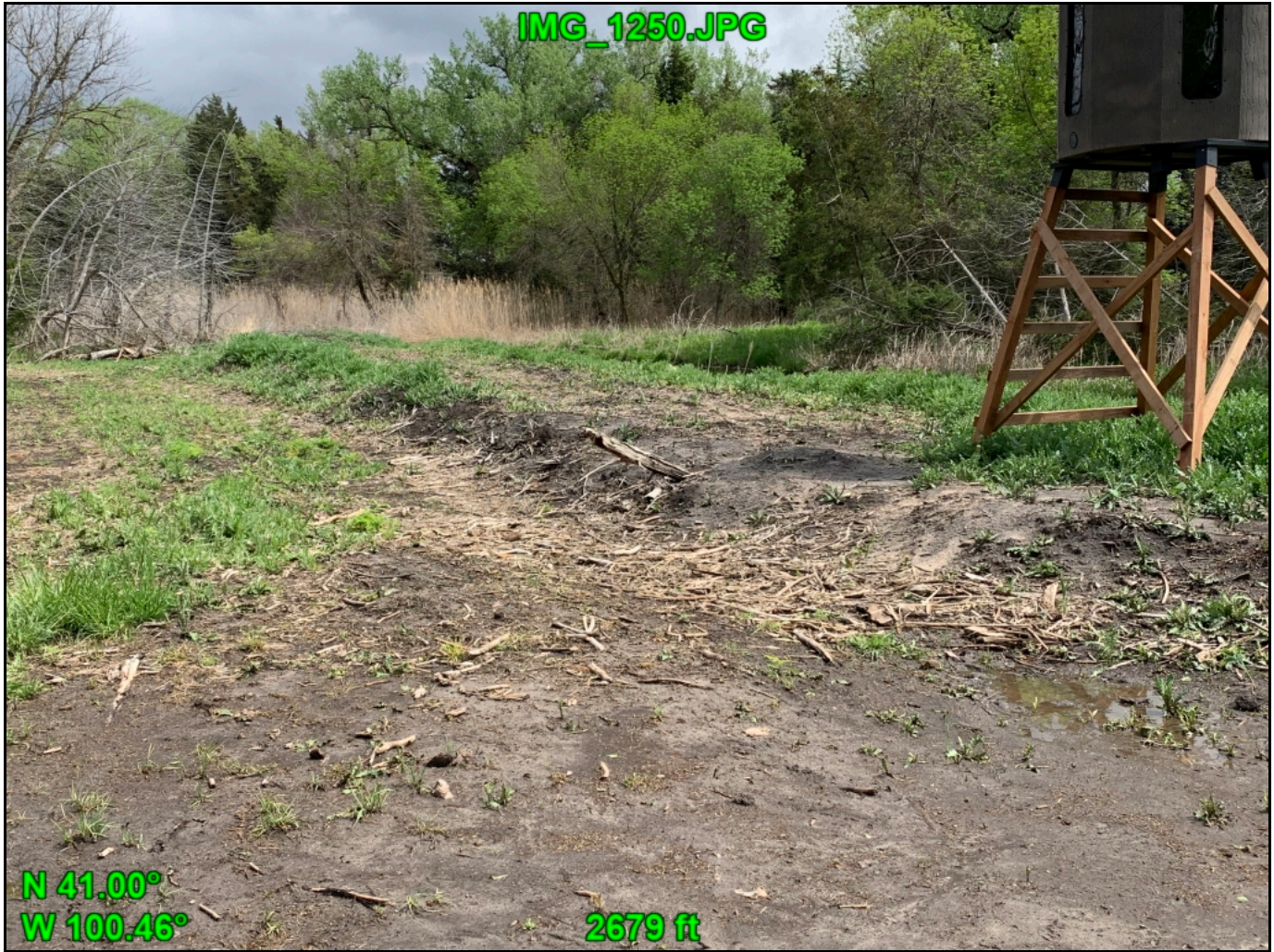
Showing berm as above.
