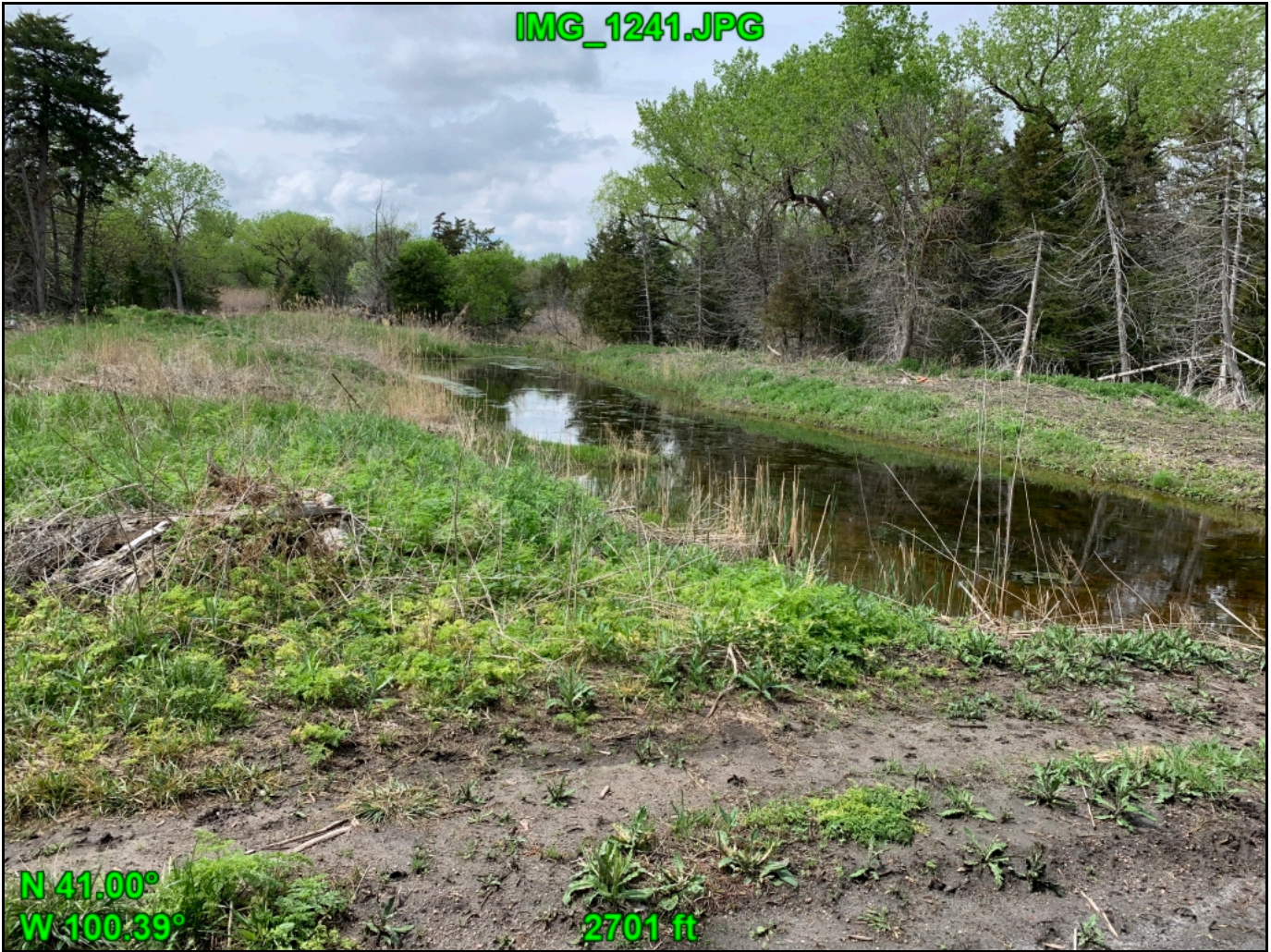
Photo taken facing west showing excavated channel south of the crossing.
