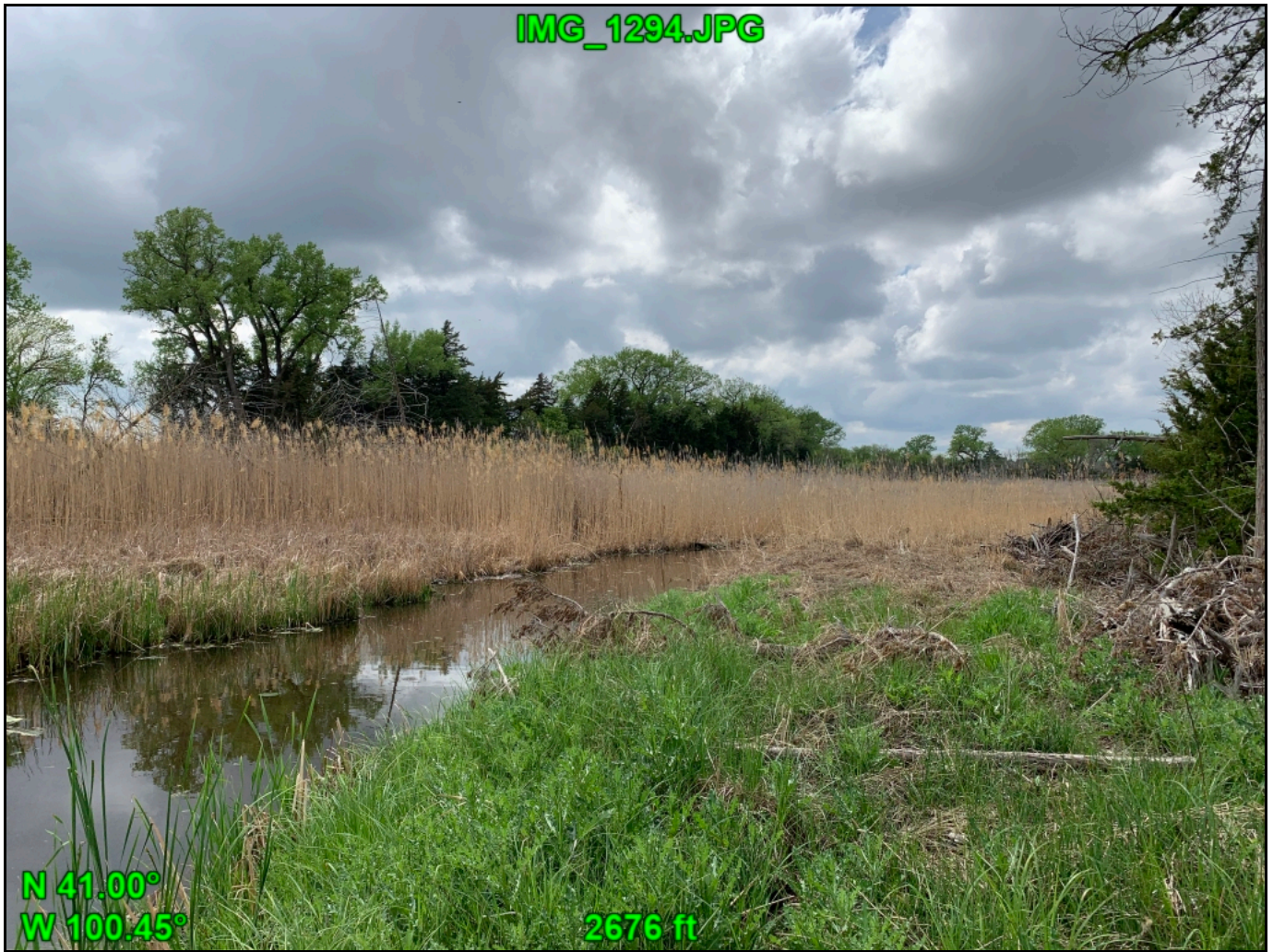
Excavated channel east of crossing 3.
