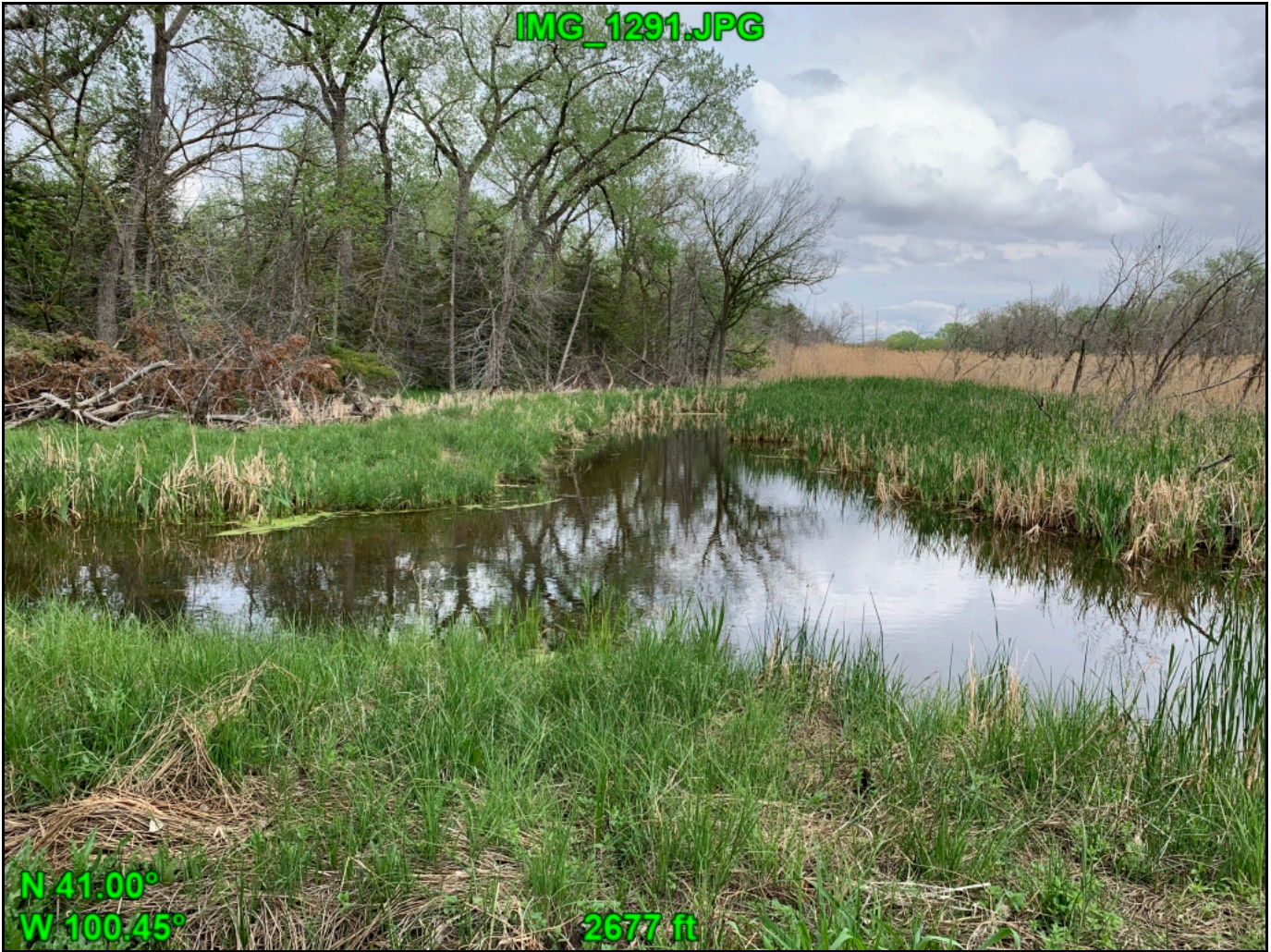
Excavation east of crossings 3 and 4.
