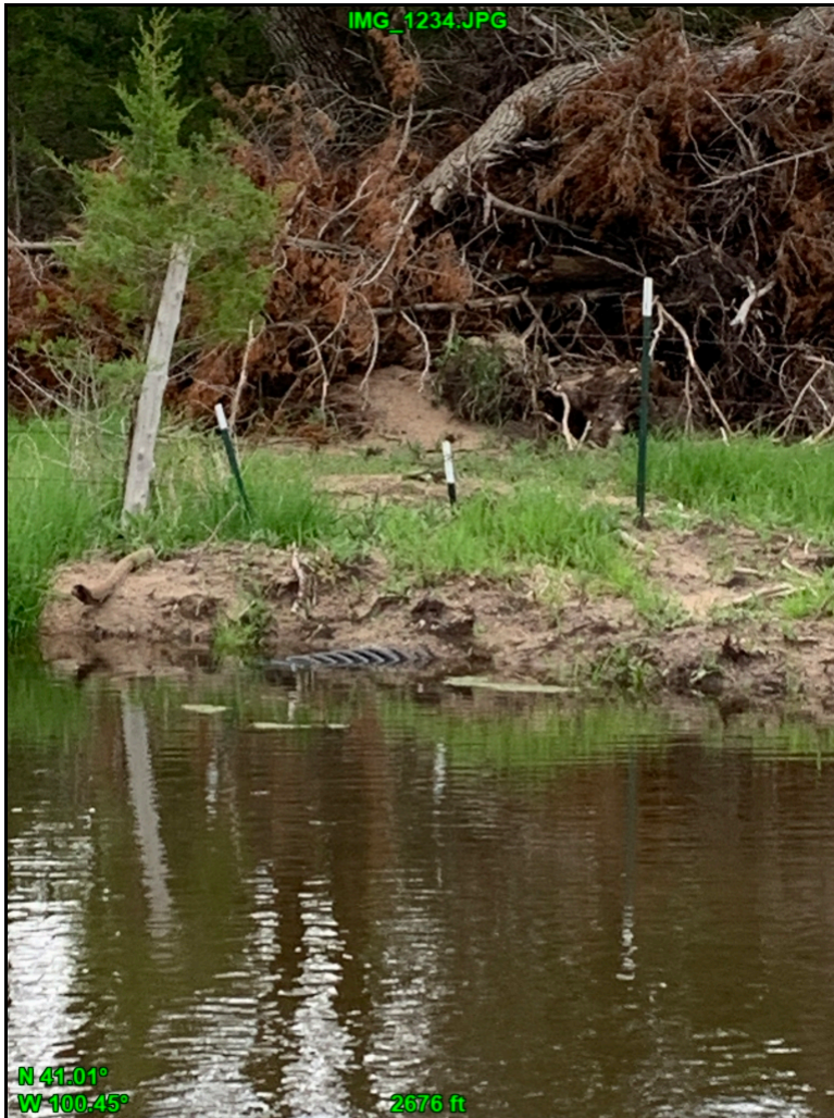
Photo showing the culvert installed below the berm.
