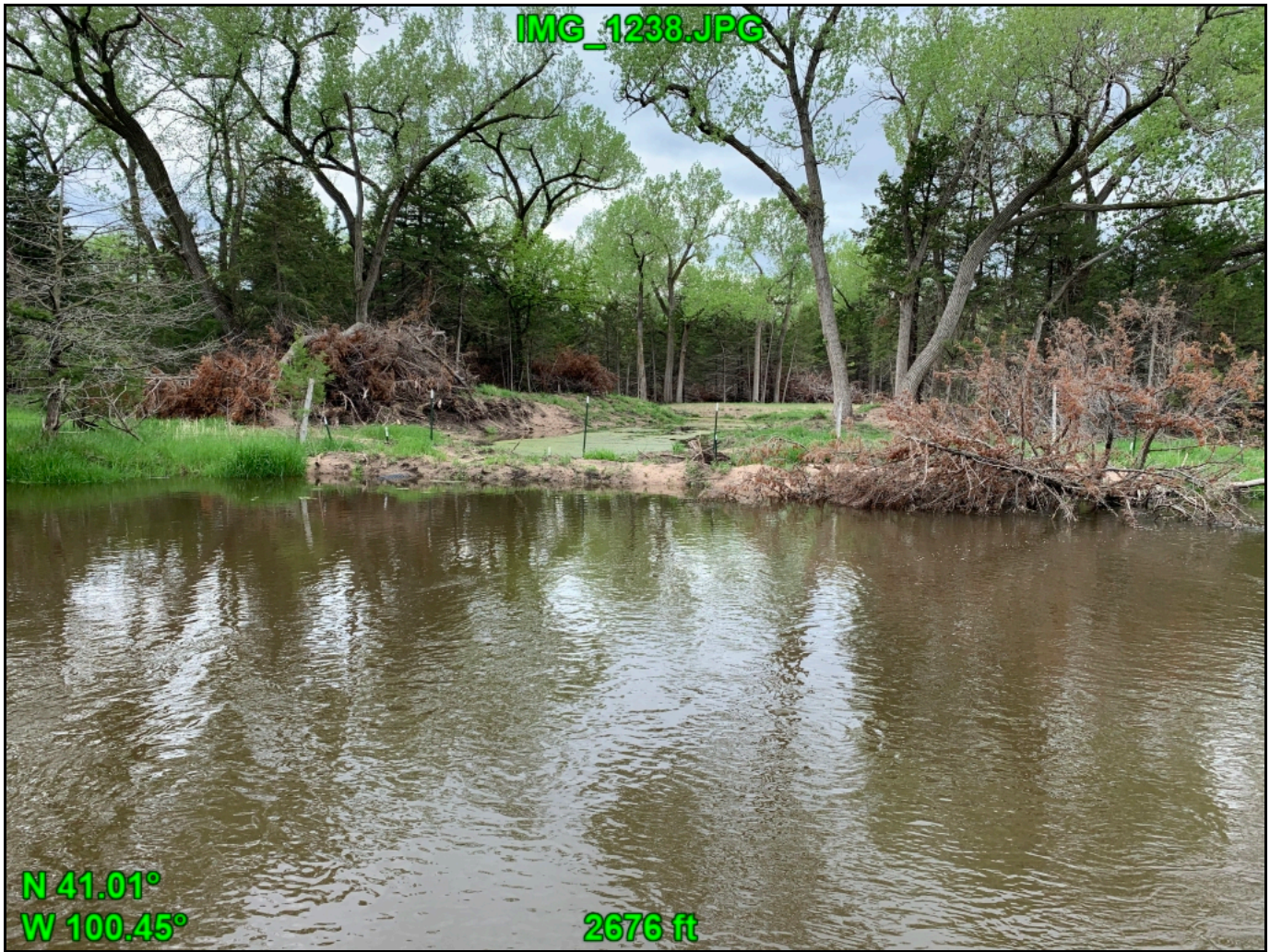
Photo taken from the north side of the channel facing south. The photo shows the area excavated behind the fence line and the berm installed between the channel and the newly excavated channel. There is a plastic culvert (about 24-inch) installed connecting the excavated area to the channel.
