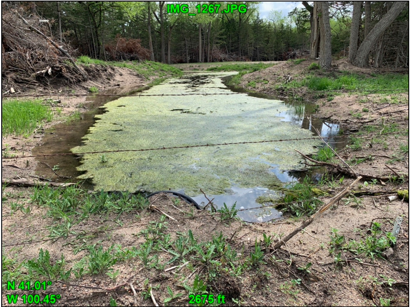
Berm and excavated channel.
