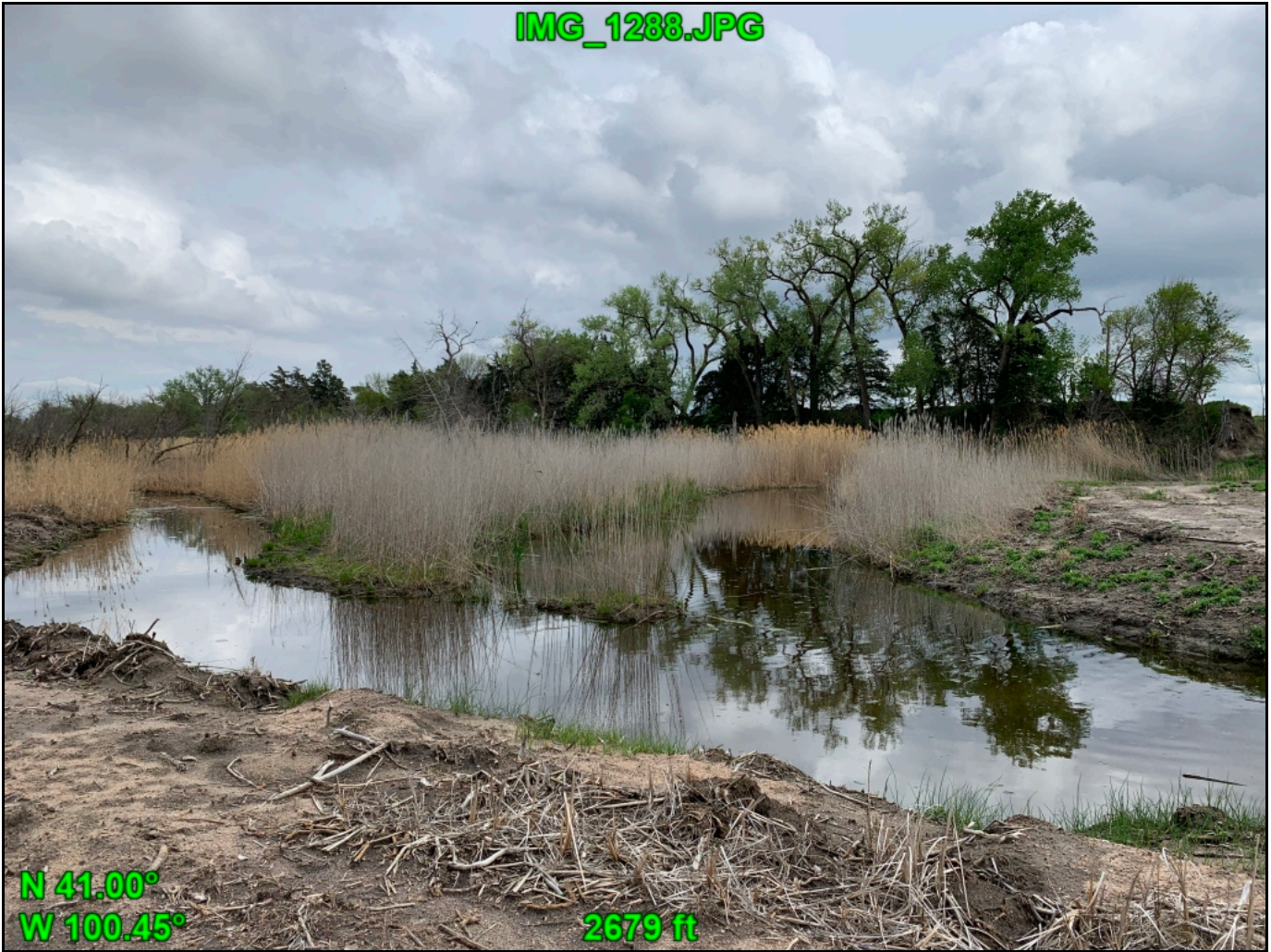
Excavated channels east of crossing 4.
