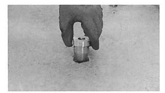
Figure 3. Installing the Drilling Guide.
