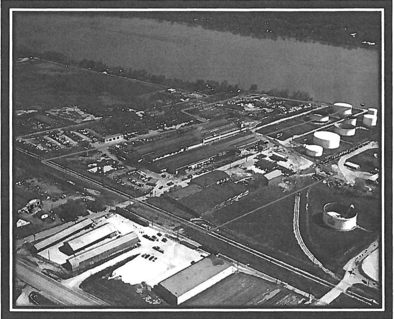
Figure 1 – Sivyer Steel Corporation, Bettendorf, Iowa
