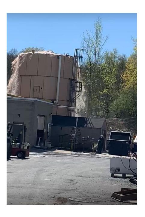
2. From IMG\_1300 Untreated process wastewater from EQ tank overflowing.
