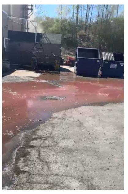
5. From Video IMG\_1300 – May 9, 2022, Untreated process wastewater from EQ tank overflowing and wastewater flowing into and being hosed into catch basin
