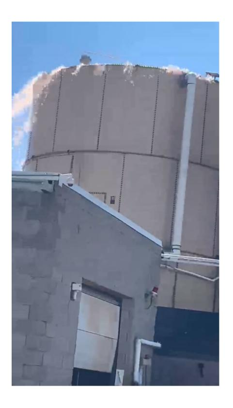
3. From Video IMG\_1300 – May 9, 2022, Untreated process wastewater from EQ tank overflowing flowing towards storm drain/catch basin.
