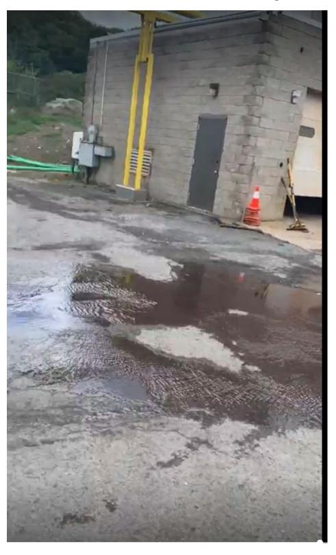
4. Wet well overflow wastewater entering storm inlet.
