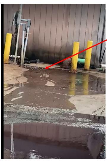
KJ Poultry Treated process wastewater wet well overflowing.
