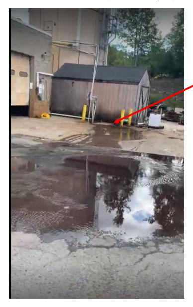
KJ Poultry Treated process wastewater wet well overflowing.
