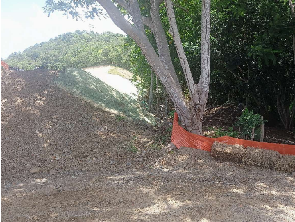
Southeast corner slope working with the implemented erosion control blankets.
