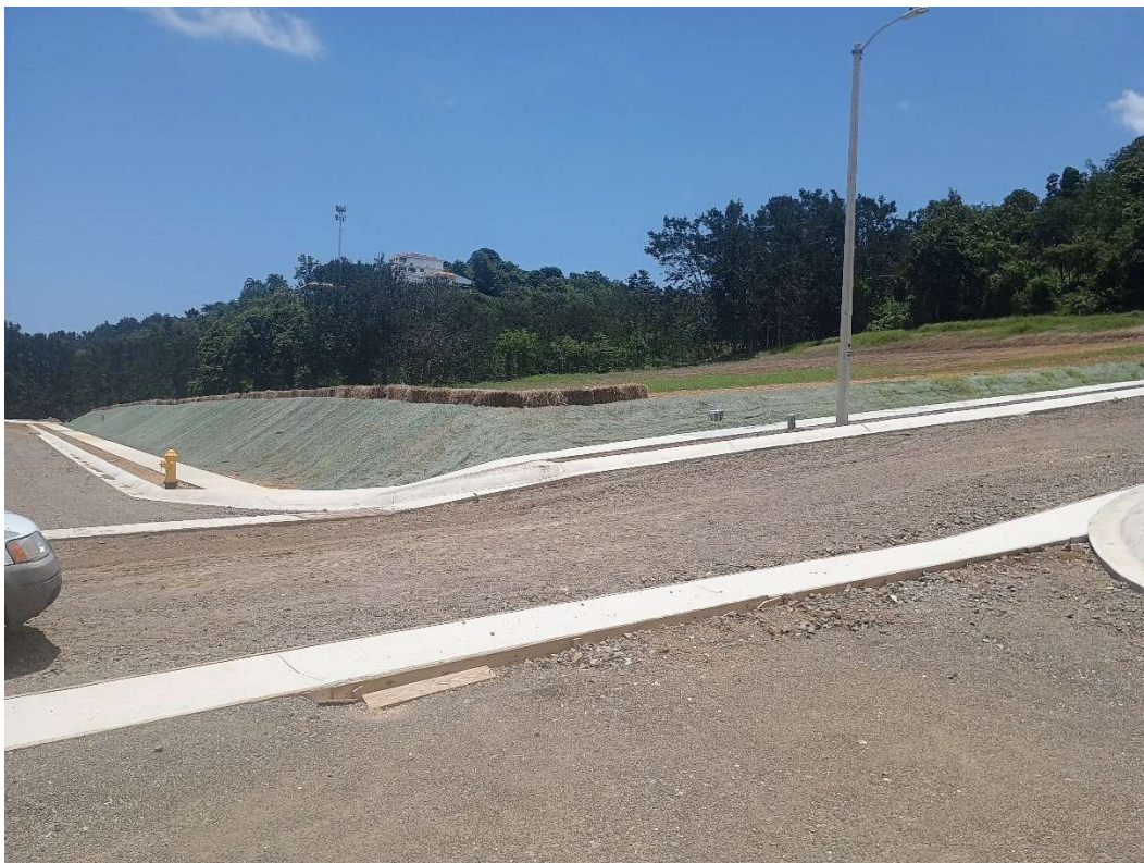
Another view of the west side of access road number 2 with erosion blankets on slopes and hay bales. Also, with temporary stabilization with gravel to prevent further erosion
