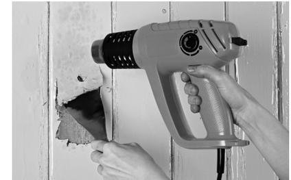
There is no way to eliminate dust, but some renovation methods make less dust than others. Contractors may choose to use various methods to minimize dust generation, including using water to mist areas before sanding or scraping; scoring paint before separating components; and prying and pulling apart components instead of breaking them.
