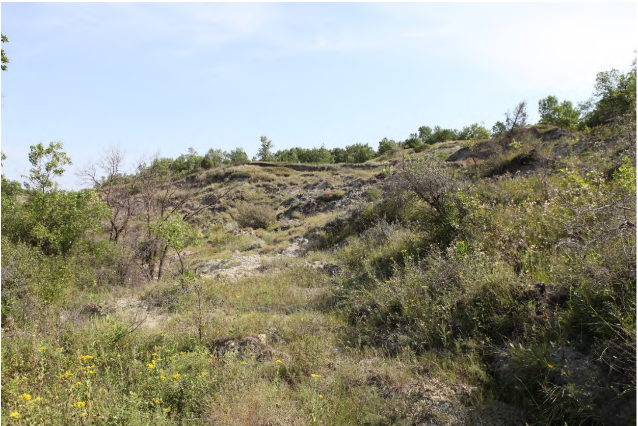
Representative landslide feature on the east side of unnamed drainage near Coulee Start (S6) — looking north/northeast.
