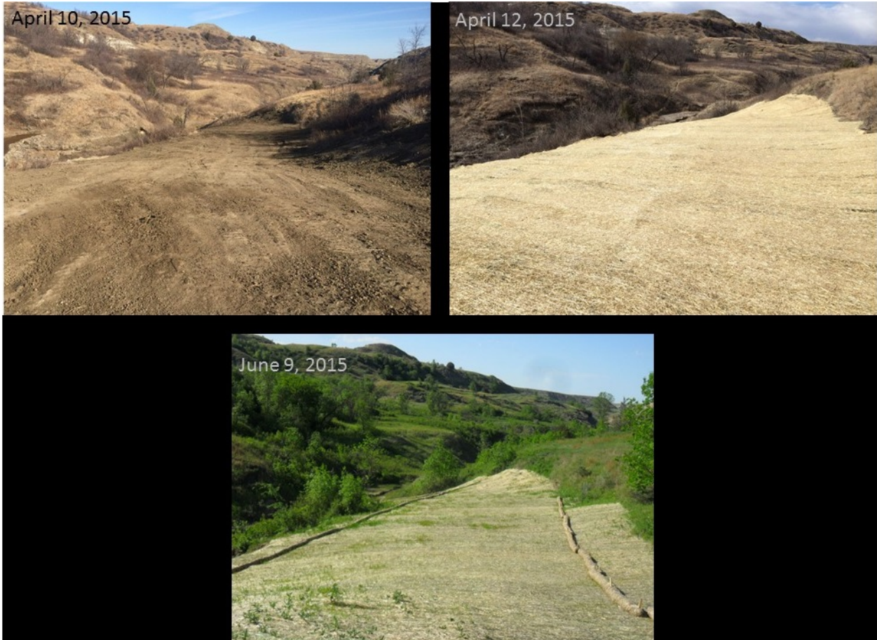
Area D, above pumpout pond; looking north.
