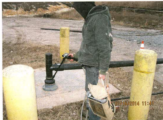
Exhibit 20 - Cell 3 Primary Pump Station 1-16-14
