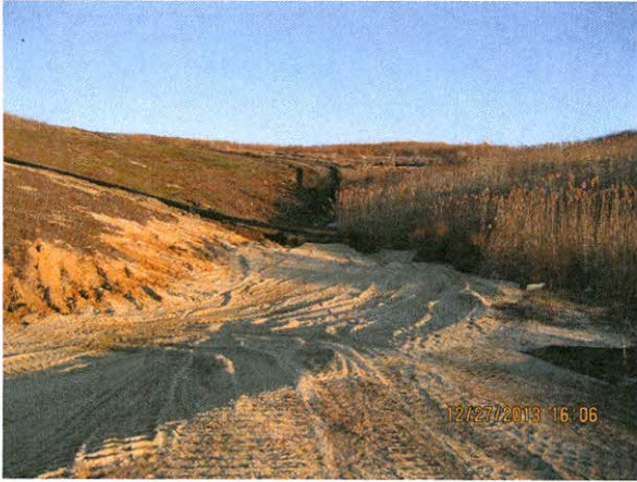
Exhibit 10 - Crevasse Between Cells 3 and 10 12-27-13
