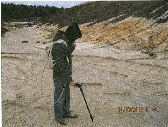
Exhibit 22 - Crevasse Between Cells 3 and 10 1-16-14
