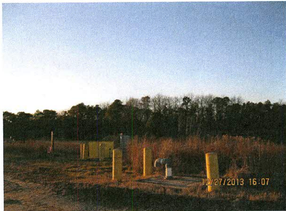
Exhibit 8 - Cell 3 Primary Pump Station 12-27-13
