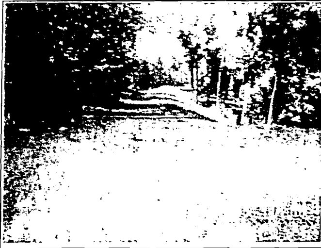
IMAGE # 9 LOCATION: SWPPP Area 3 DESCRIPTION: Grading and earthwork ACTION REQUIRED: Some ground hydroseeded - no action; seed & stabilize disturbed area exposed 14+ days.
