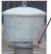
For elevated tanks, having fewer than 8 inches from the bottom of the #24 mesh to a horizontal surface will trigger a significant deficiency The vent must have a watertight cover that extends down to the bottom of the #24 mesh screen. The cover will prevent the entry of rain and snow as well as minimize the entry of dust.
