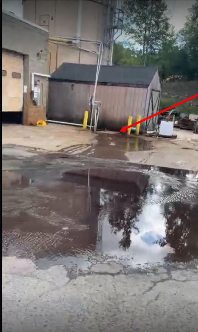
KJ Poultry Treated process wastewater wet well overflowing.
