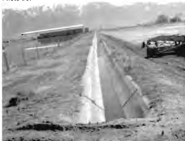
Concrete channel along the south side of the evaporation pond used to drain and divert pond water to fields owned by facility owners. Pond water not analyzed for nutrient content.
