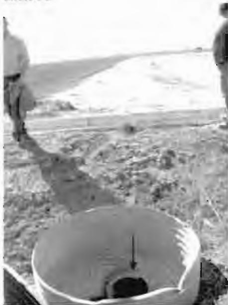
There are drain pipes in the fields (top of photo) that capture excess water to this outfall (arrow) (in same metal ring in Photos 36 and 37) that contains the drain to the slough.
