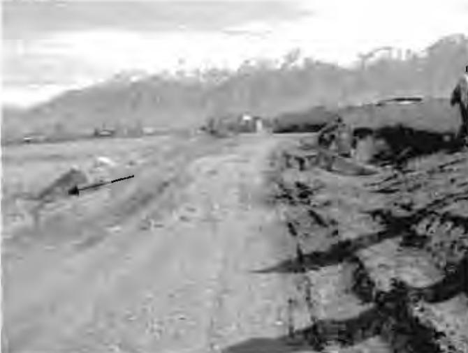
Looking northeast from the same location as Photo 22. Note the breach in the facility berm (arrow). The facility believes that storm water from the access road (seen in Photo 22) has not be contaminated with process water and could therefore drain into the slough.
