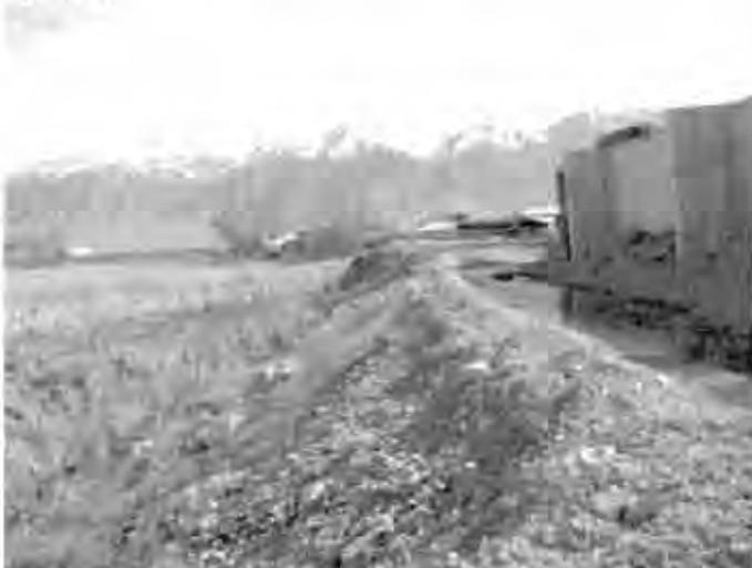
Surface drainage going to pump area. Water is from broken water line that is under repair. Photo shows water flow pattern.
