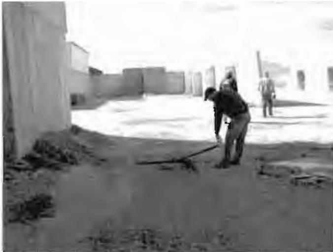
Drain behind hay shed. When there is heavy precipitation, the cover is lifted to allow the area to drain. This is a heavily tracked area. Cover is used to minimize the debris that may enter the drain.
