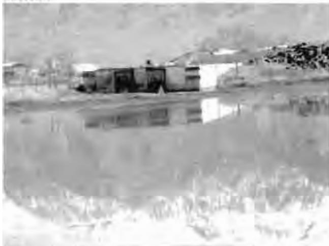
Looking north across evaporation pond at the separation cell. Process water from pump in Photo 18 goes to these cells. Facility indicated it used the water mark (purple arrow) on the right cell wall. If pond water is above this water mark, there is 6" of freeboard. If pond water is right below the weeping walls (red arrow) there is no freeboard in the pond.
