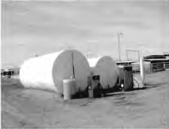
Diesel tanks: 6000 gallons is in use; 2000 gallon has rust and not in use.
