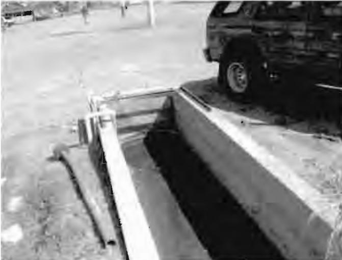
Close-up of end of concrete channel. Water flows in an underground pipe to a pump station approximately 150 feet to the north. Photos of the pump are in Photos 43 and 44
