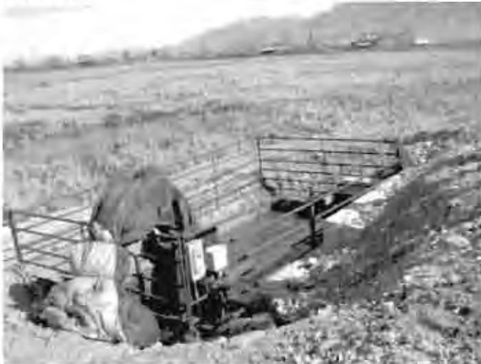
Pump area. Drains flow to this site. Wastewater is pumped to evaporation pond.
