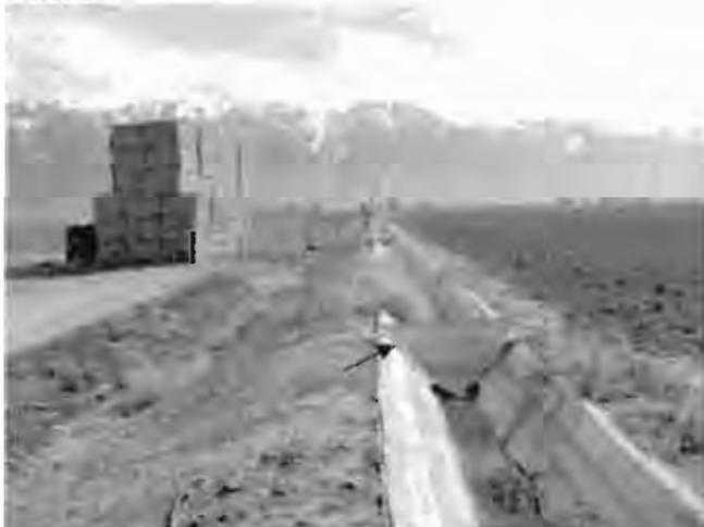
Looking east, this concrete channel connects to the channel in Photo 30. From this channel water is distributed to the facility owners' fields. The facility representative indicated the metal baffle (arrow) was installed to stop water from continuing east. Water was observed beyond the metal baffle.
